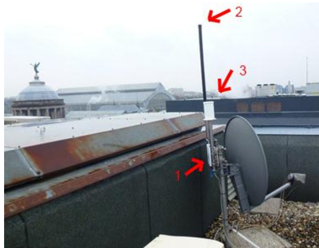
Figure 14 – Location of the RFeye (1) and antennas (2,3) at the Brussels measurement station
