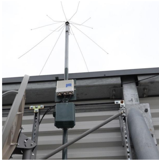
Figure 9 – Mounting location of the antenna for the Seattle measurement station
